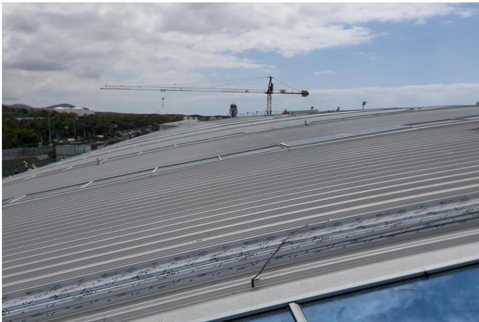
*Photo of the construction phase – The Kalzip sheets have already been installed.*
