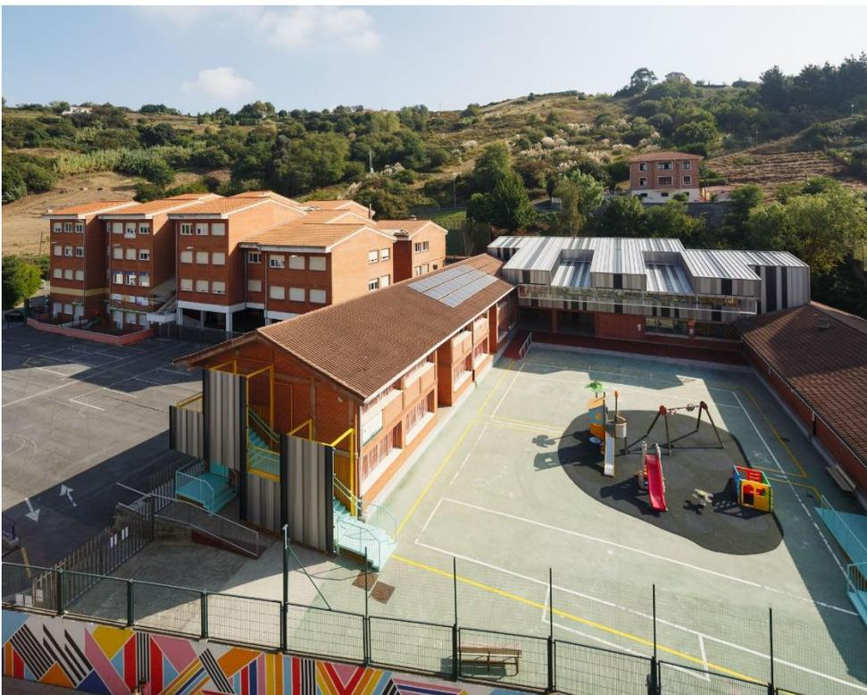
*Three RAL colours were used for the roof and the façade. Perforated Kalzip profiled sheets were also installed in the front part of the building.*
