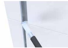
1. To remove an individual panel from the façade, the panel above it must first be unclicked at it lower edge. When using the panel removing tool with round grip, the panle may need to be slid to the one side to create sufficient space to insert the tool into the vertical joint. Insert wedges and unlock the fixed point clamp. Slide the panel to the side and relock the fixed point clamp. Remove the wedges.
