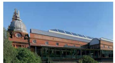
Manufactured inside the main hall, the Kalzip® sheets were then transported up to roof level for installation. The external face of the Kalzip® sheets has a highly durable AluPlusPatina finish providing a traditional appearance that blends sympathetically with the rest of the building and its surroundings.
