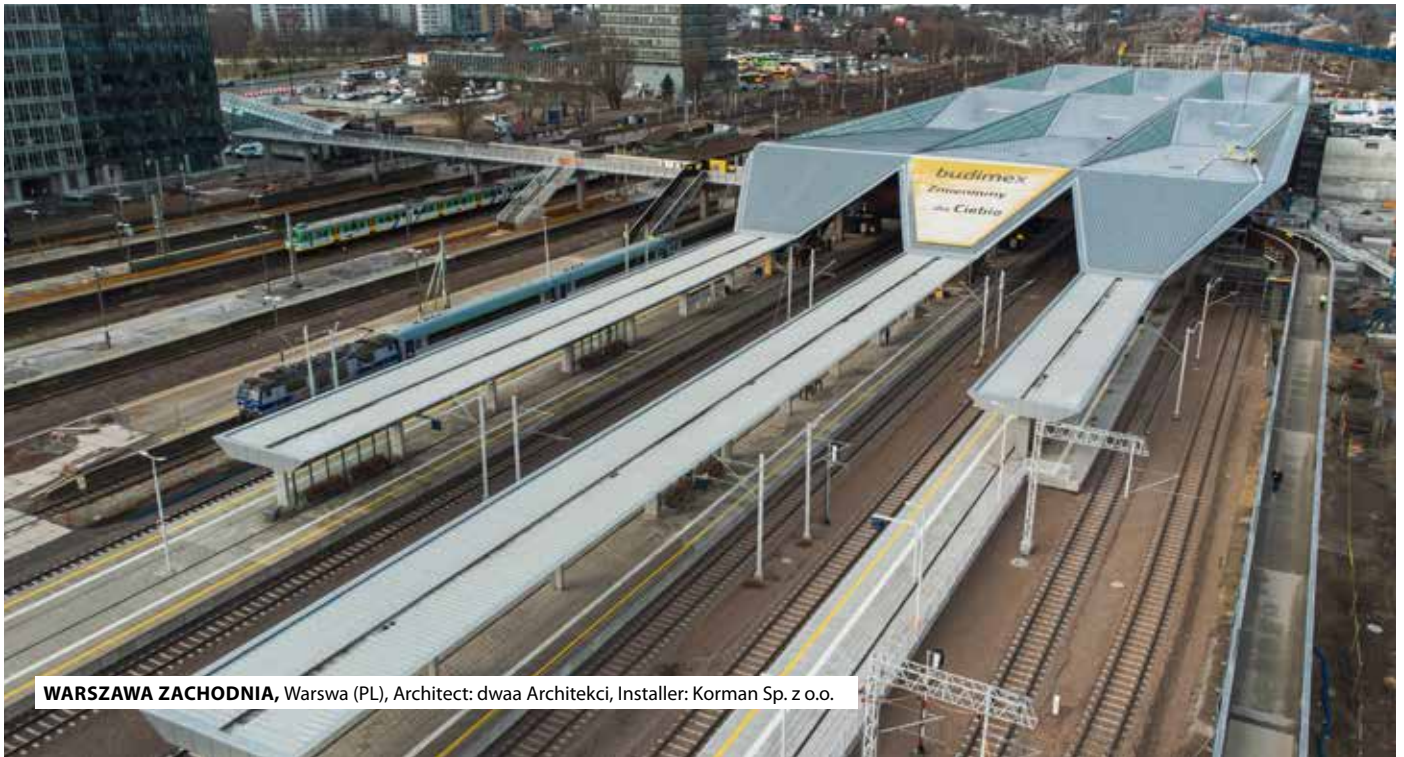
Kalzip standing seam on structural decking
