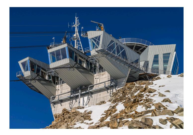
A Kalzip vapour control barrier was glued onto this. Finally, the visible exterior was finished in angled standing seam roofing, using 0.7 mm thick FalZinc<sup>®</sup> aluminium sheets. In total, around 7,000 m<sup>2</sup> of FalZinc<sup>®</sup> aluminium profiles were installed on the project.
