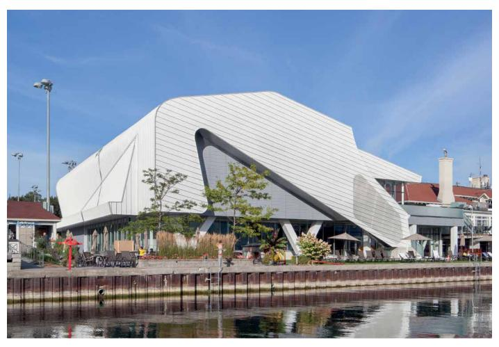
"We were really excited by the ability of Kalzip® to produce extremely long cladding sheets, each capable of being shaped to the precise profile of the building. This enabled us to design an elegant watertight structure able to withstand high wind loading and extreme temperatures whilst at the same time providing a clean, continuous and uninterrupted roofline that rolls seamlessly into the walls, creating a beautifully flowing building envelope."
