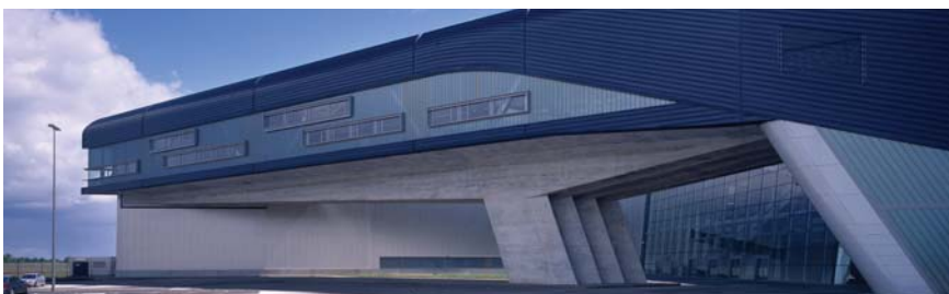
Project: BMW Central Building, Leipzig, Germany Architect: Zaha Hadid, Patrick Schumacher
