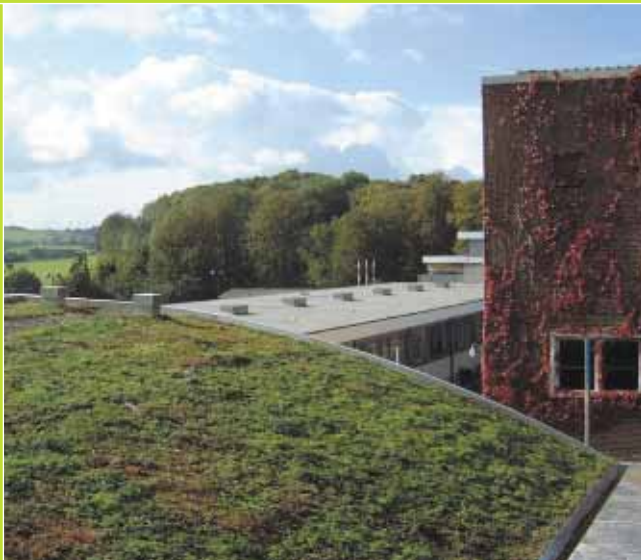
House for the Future, Museum of Welsh Life, St Fagans. Sedum mat installation
