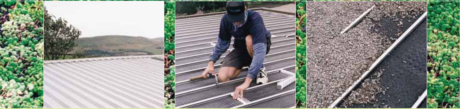
Stucco embossed Kalzip roof
