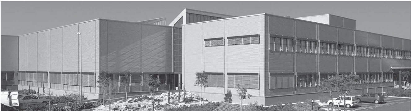
Bosch industrial plant Bari/Italy, Robert Bosch GmbH
